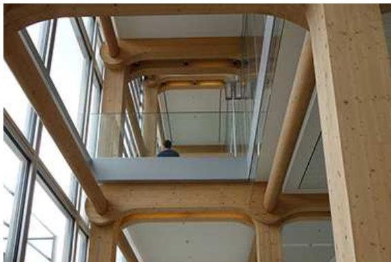
FIG.6. Tamedia office building in Zurich from 2013, built with laminated timber beams with extensive use of CNC-machines, Shigeru Ban architects (photographs of the case study buildings by the author)
