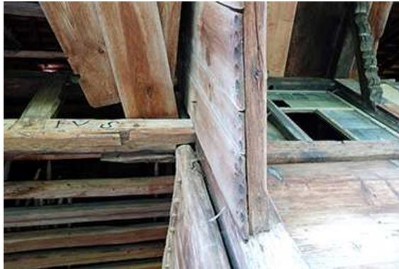
FIG.3. The case study buildings: Vernacular farmhouse in CH-Birrwil from 1692, timber frame with infill of wooden panels and rich ornamentation. (photographs of the case study buildings by the author)
