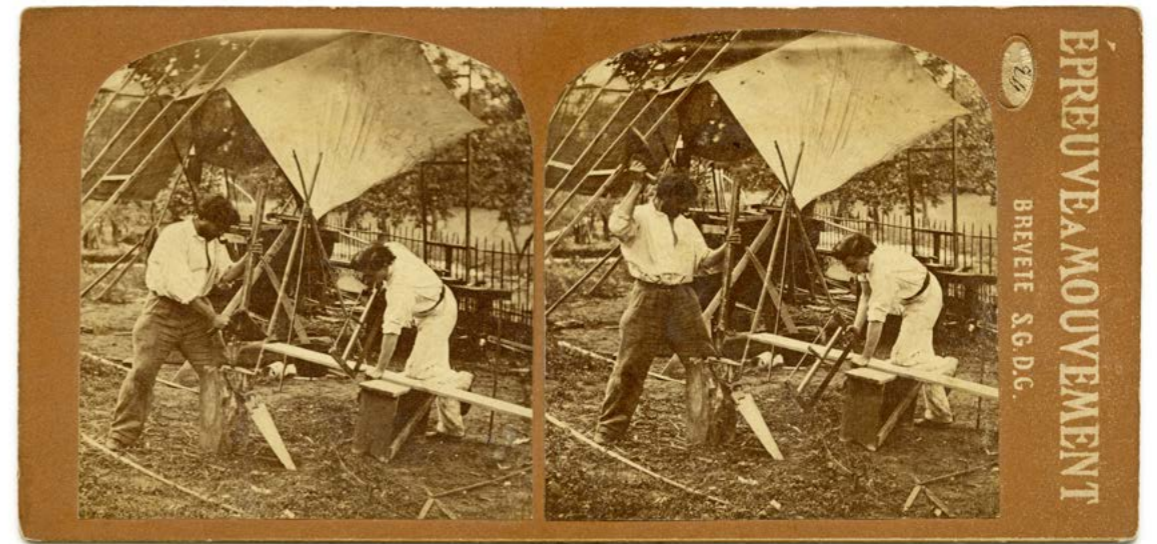
Figure 7. Furne and Tournier. "Epreuve à Mouvement". No. 24. Man sawing and other man whittling down the end of a stake to a sharp point with an axe.
